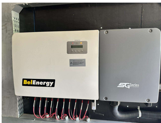
Figura 12 - Inversor Solis 110kW-5G
